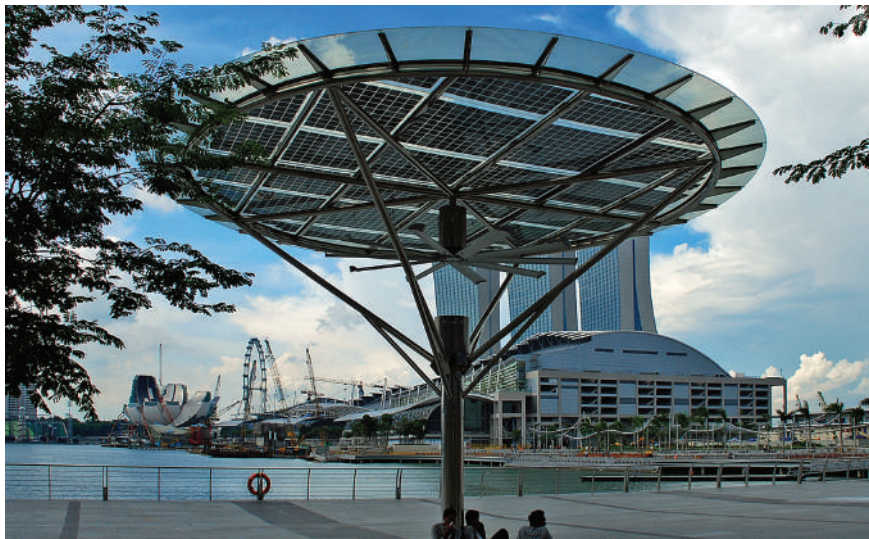
Solar-Powered Breeze Shelters in Singapore. Photo by Choo Yut Shing (Permission under CC BY-NC-SA 2.0). Along the Marina Boulevard, these pavilions are made of glass and stainless steel, and feature large fans.
