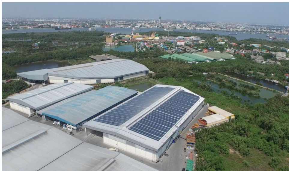
998 kW System at the CRC Wharf, Credit: Photon Power
